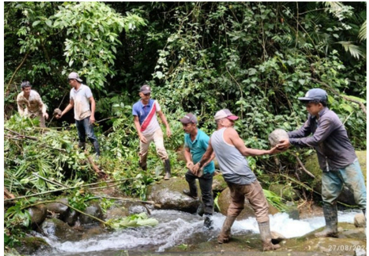
Community members passing boulders to build water capture
